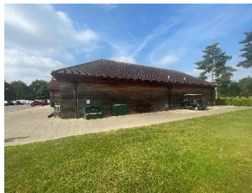
Side of the Clubhouse
