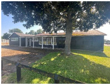
Slough Town Clubhouse before Demolition
